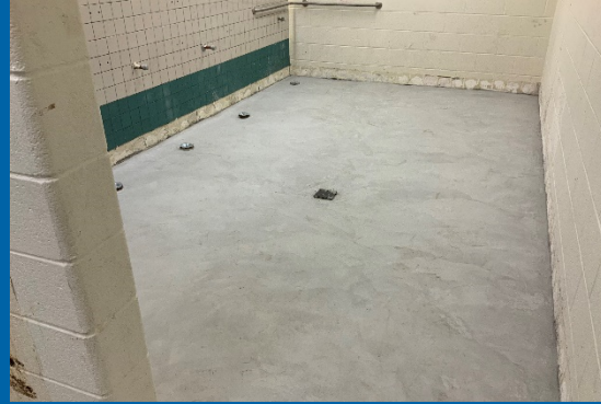
Poured Topping Slab in Restrooms
